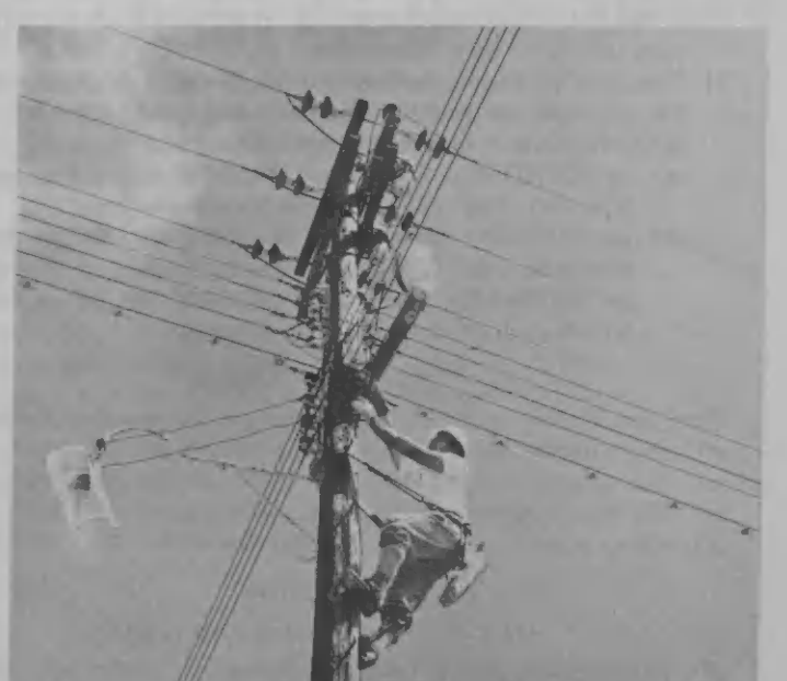
WHEN CLIMBING poles, electricians are well protected through the use of safety belt and other equipment. ORA TA subi, palu, electricistanan ta bon protehá door di usa faha di seguridad y otro equipo.
